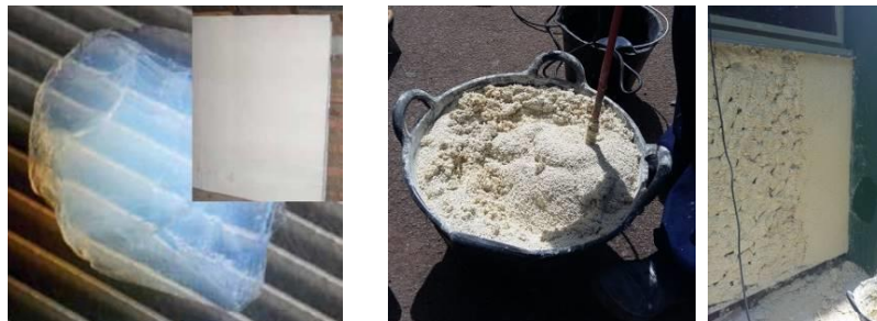
Figure 3. Image of aerogel and aerogel mortar insulation
