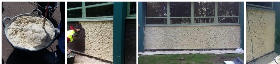
Figure 12: Installation of the aerogel mortar
