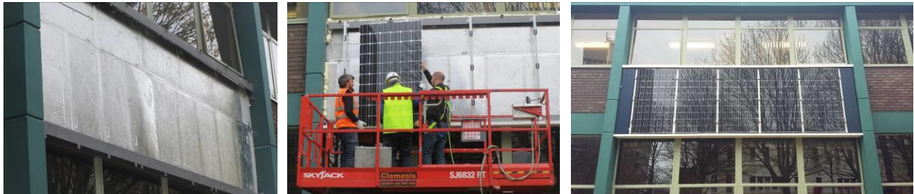
Figure 11. Installation of the ventilated façade
