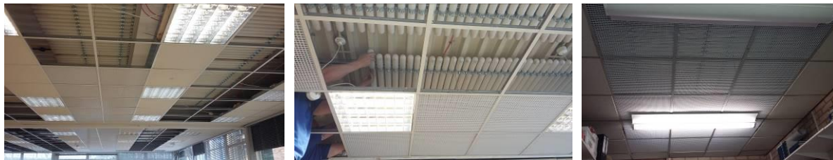
Figure 9: Installation of the PCM tubes
